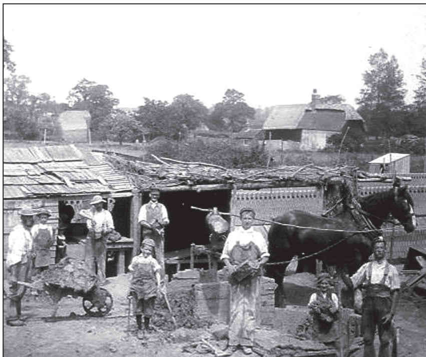
Plumpton Cox's Brickyard
